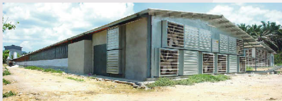
TUNNEL VENTILATION HOUSE
